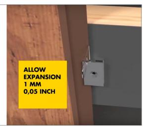
• Place the remainder of the cladding planks up to the corner or edge.
