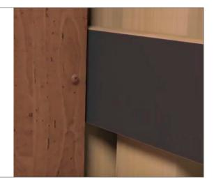
• If a roof trim is used to finish your installation, leave a 5mm gap between the top of the cladding planks and the trim.
